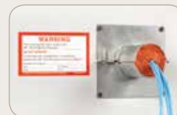
Installation of putty and application of identification label completes pass-through firestop. Putty holds cables in position, helping to prevent cable slippage and movement.
